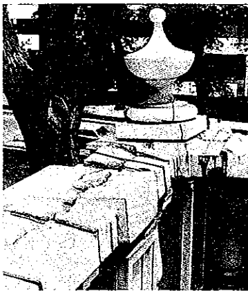
Figure 8. Deterioration of Exposed Detailing. Exposed or freestanding terra-cotta detailing (parapets, urns, balusters, etc.) have traditionally been subject to the most severe vicissitudes of deterioration as a result of freezing temperatures and water. (Colorado State Historic Preservation Office)
